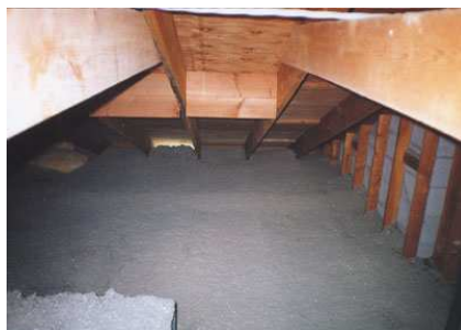
View of blown cellulose insulation.
